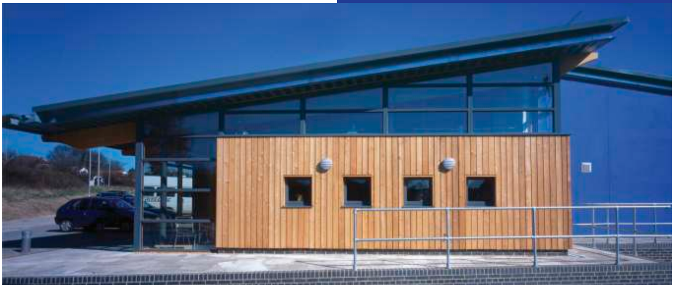
TOP: Resource Centre, Earley (Jessop & Cook Architects Ltd)
