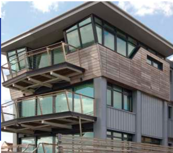
TOP: Resource Centre, Earley (Jessop & Cook Architects Ltd)
