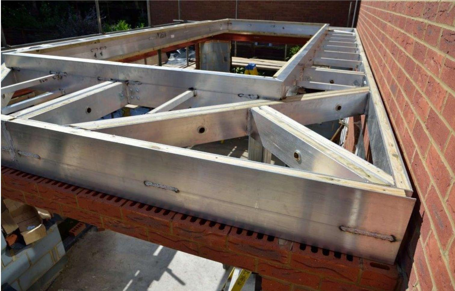
A typical 7m x 5m **iX250** orangery deck can be lifted into place and connections secured in around 2 hours
