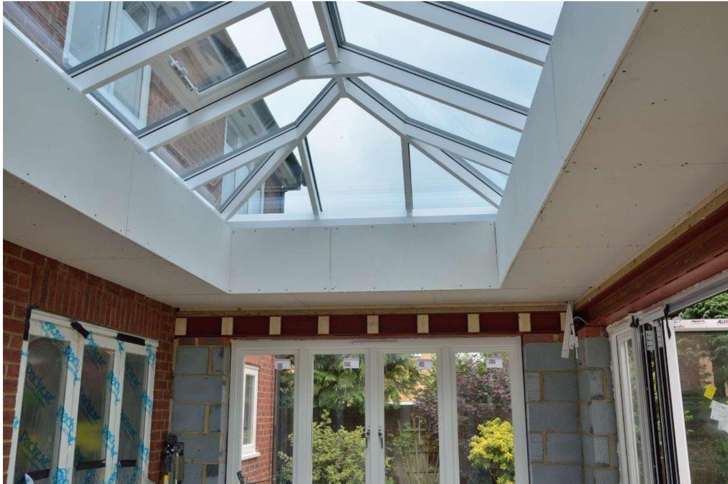
After the glazed lantern has been installed, the internal deck can be plaster boarded
