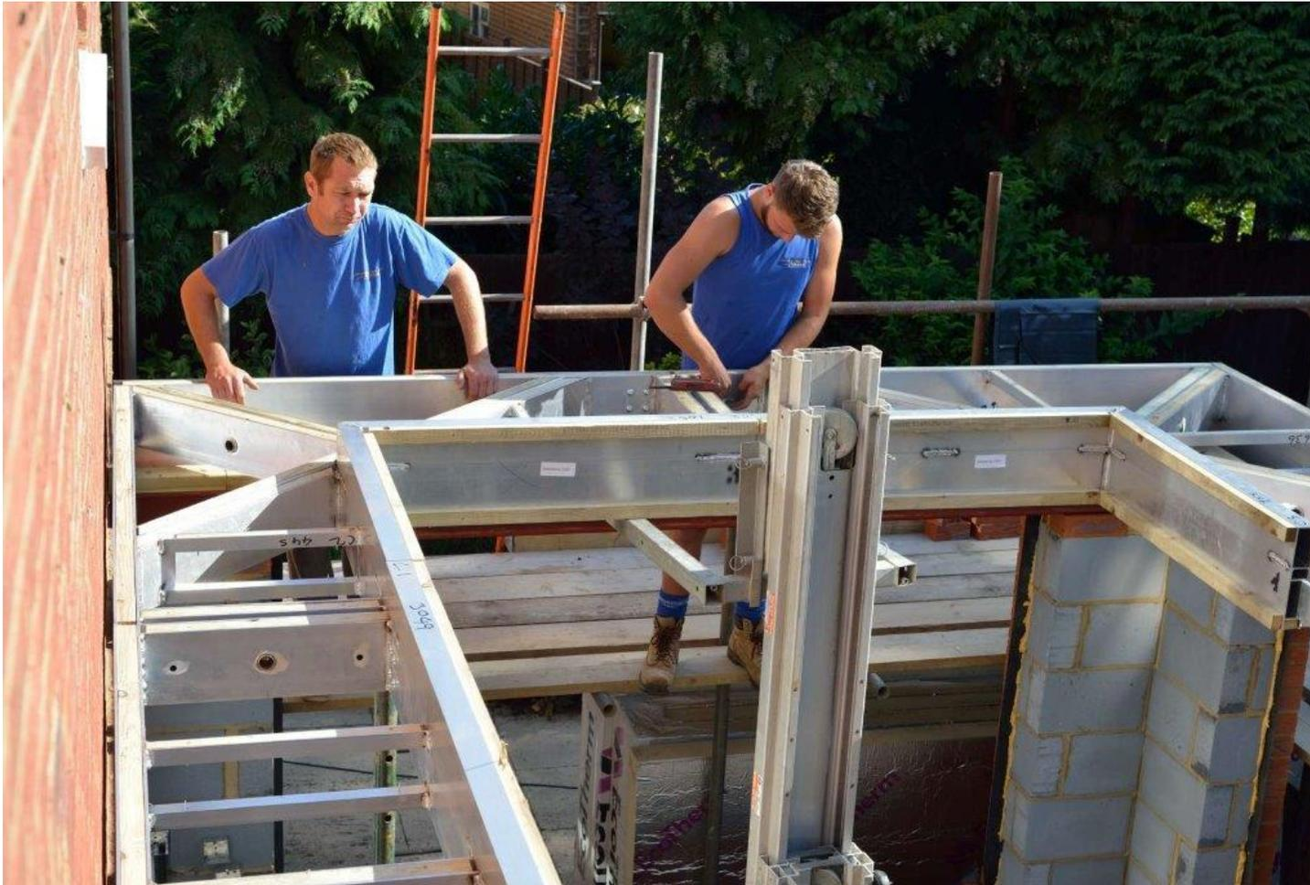
**iX250** prefabricated sections can be lifted into place quickly and easily with just two installers
