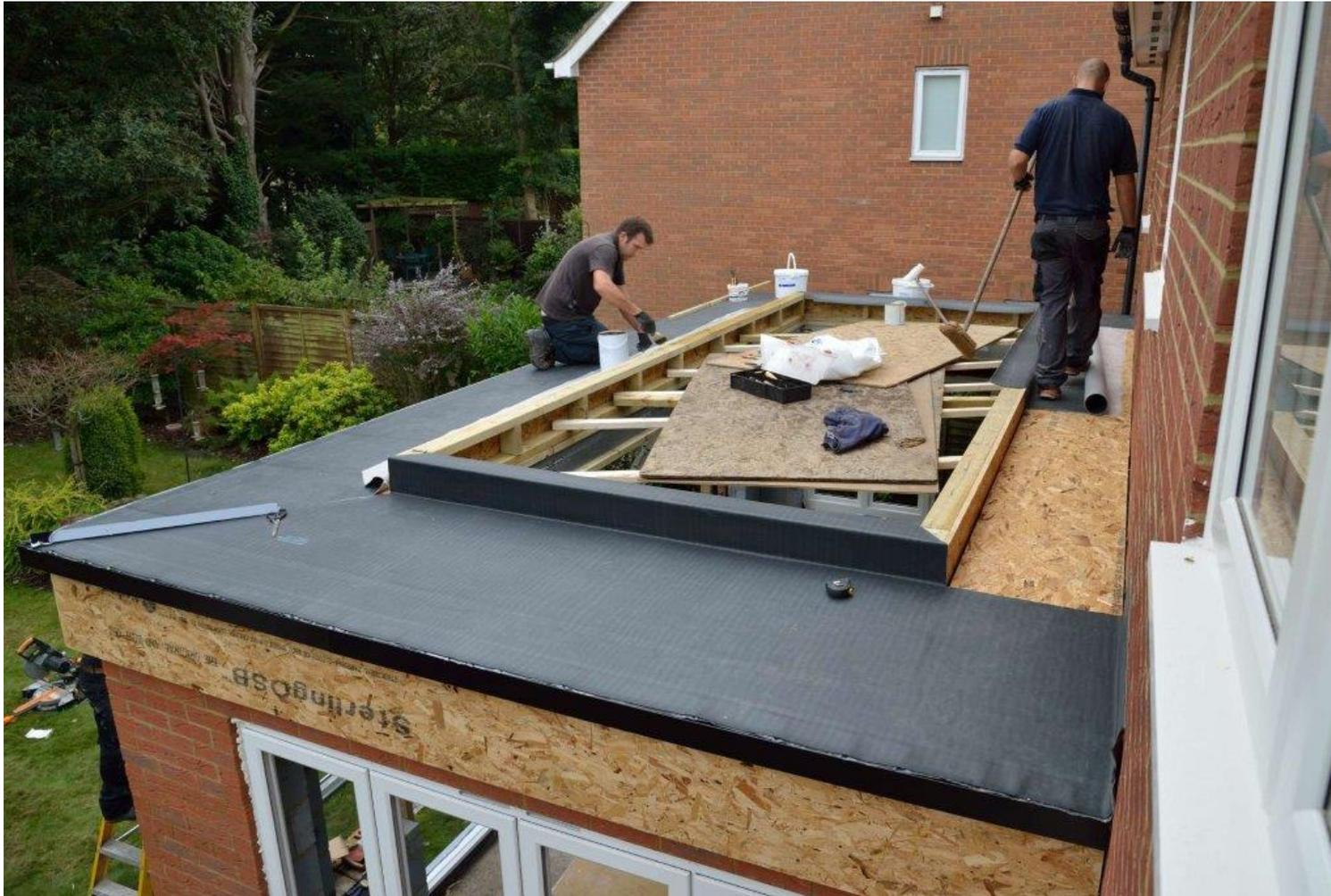
Once insulation and decking boards have been fixed into place the perimeter roof section can have the specified covering applied
