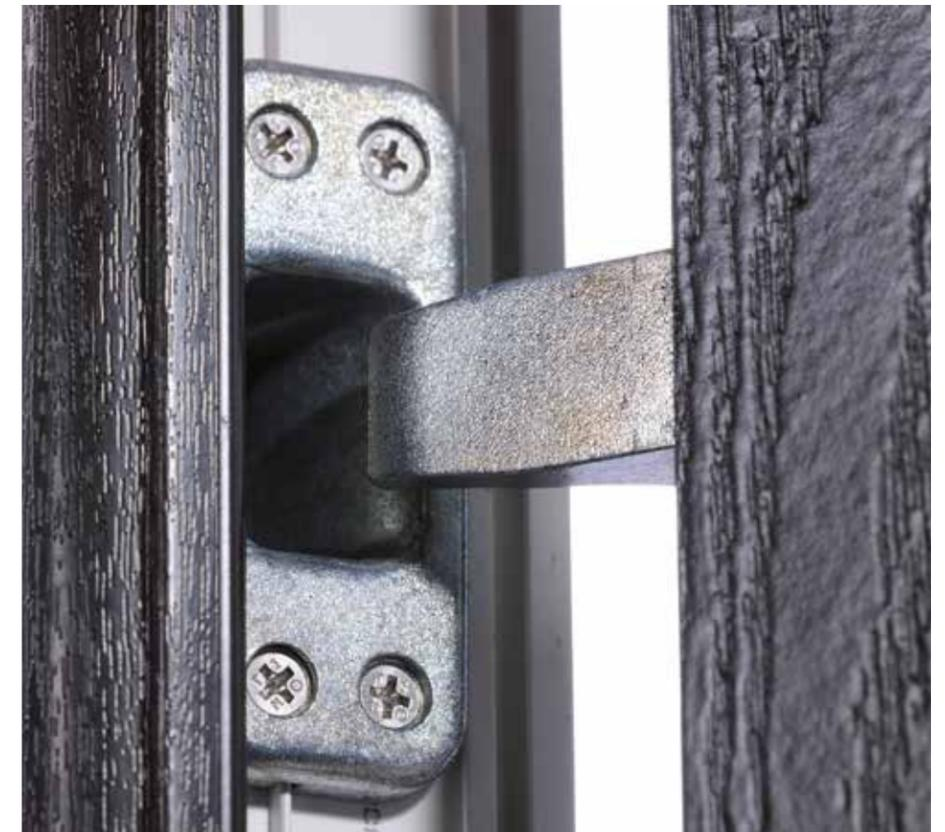
Multi-point Yale locking system features two rollers, three hooks, two deadbolts and a latch. It secures the door from top to bottom.
